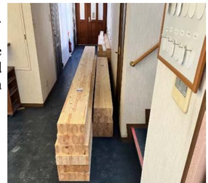
New Posts and Beams
